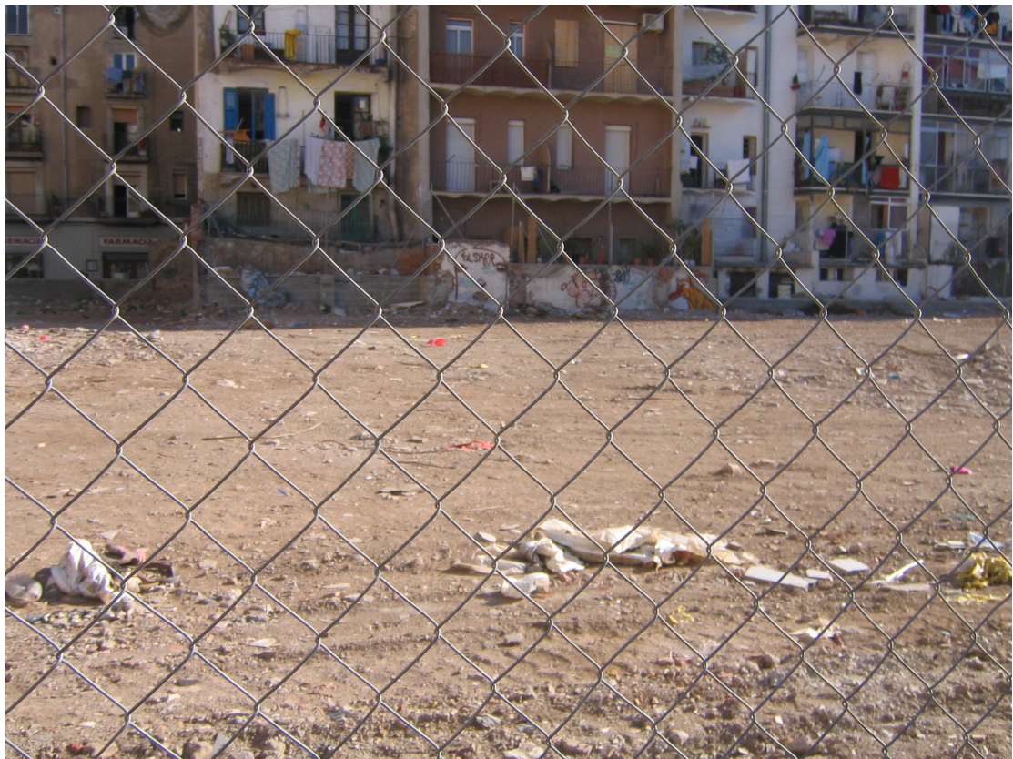
Demolition is the only solution in some areas, which are 'too far gone'.
