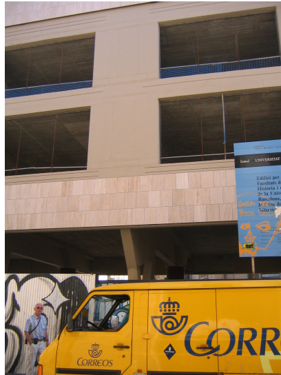
Changes and construction are still apparent around the cultural centre. Opposite is a construction site, where they are planning to build a library and university of geography, history and philosophy.
