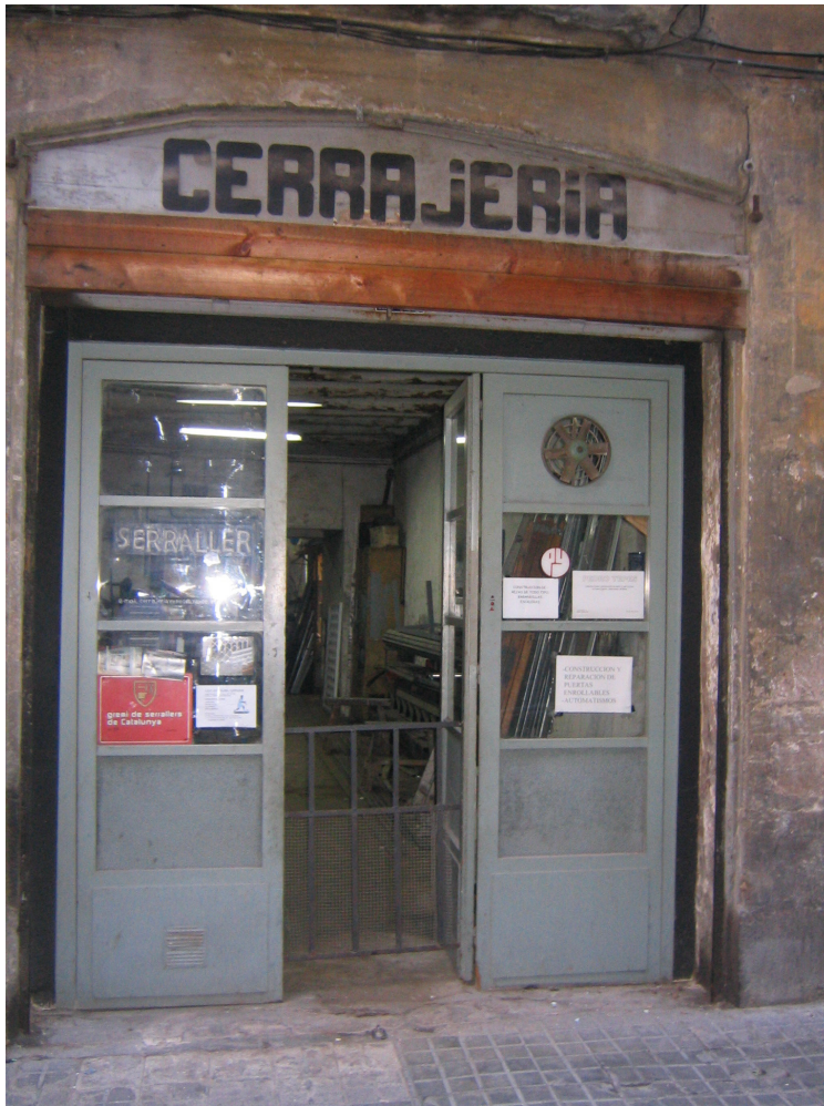
Old workshops indicate the local and traditional aspect of the area.
